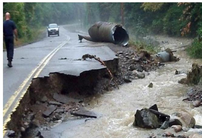
Figure 1: Damage to Highway 552 in northeastern Ontario after a heavy rain event (CBC News, 2013)
