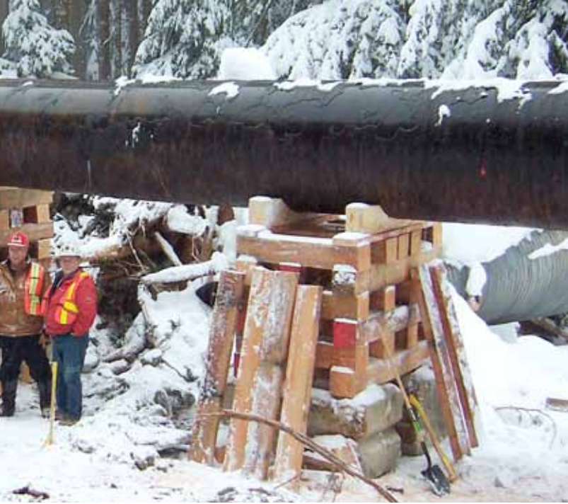
Figure 7 | Repair of damaged hydropower penstock footings
