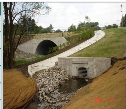
New overland flow system for Black Creek in Toronto. This was designed to prevent flood water from accumulating on the road and to prevent it from overwhelming the culvert capacity. It was built in response to the 2005 storm that washed away sections of Finch Avenue.
